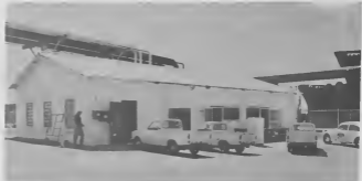
This is the Finger Pier Lunch Shelter which serves as a temporary "haven" for Mechanical field workers and dock personnel at lunch time.
